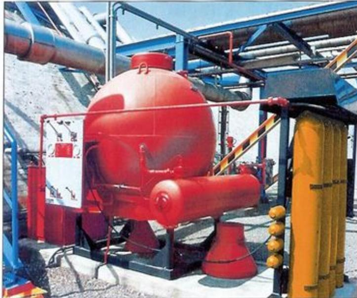
Powder extinguishing systems are fixed fire extinguishing systems for volume or object protection. The extinguishing powders are used for fires in solid, liquid and gaseous materials as well as for metal fires, i.e. for fire classes A,B,C and D.
