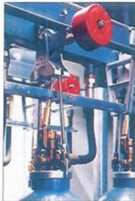
Systems are distinguished according to the way in which the extinguishing agent is stored, and in particular whether as pressurised liquid ( $CO_2$ ) or as compressed gas ( $Ar$ ,  $N_2$ ) in high pressure steel cylinders or in low pressure vessels.
